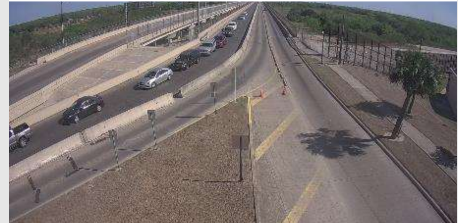
Veterans Bridge: April 25, 2020
